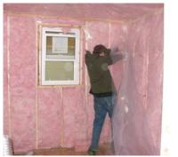
We chose to test recyclable insulation, for it would be more Eco-friendly compared to the Pink insulation. Recyclable insulation is made up from 87% cellulose recyclable fibre; it also increases your firewall by two hours of protection. You can see that the recycled insulation is just as efficient as the pink insulation. It would cost a lot less and be environmentally friendly. The R-value varies from 12-60 depending on the packing of the insulation.
